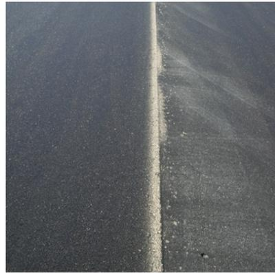
Longitudinal joint with coarse segregation.
