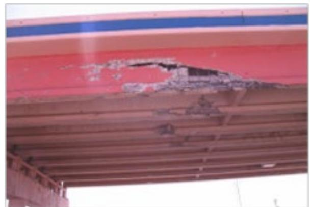
*Bridge damage from heavy load on overpass.*
