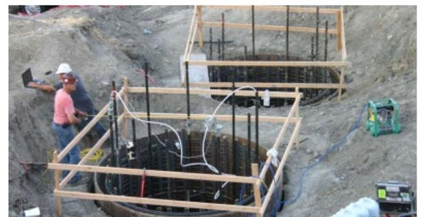
*Thermal sensors in underground tubes measure the strength of poured concrete columns.*
