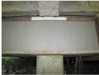
*Pile cap repaired with high-strength composites.*
