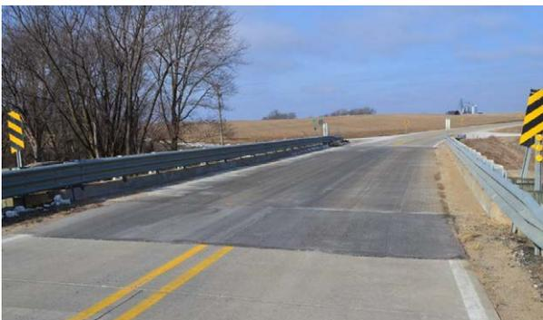
*Finished UHPC overlay on top of a bridge deck.*
