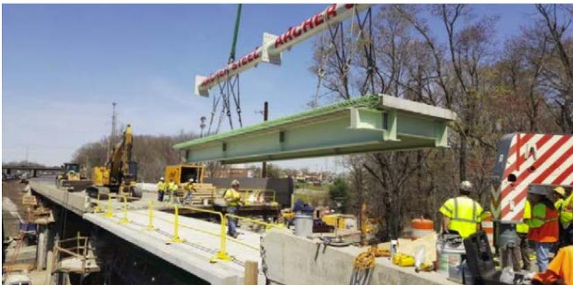
*Prefabricated wide-flange beams topped with a composite concrete deck.*
